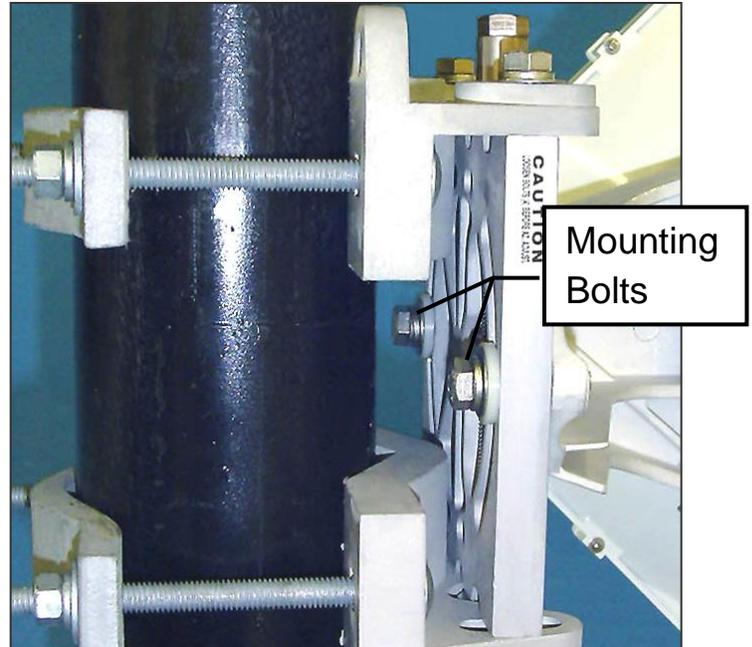
3. Tighten mounting bolts securely after elevation is set.
